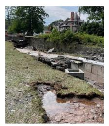
Water forces can carry large boulders and man-made structures such as this culvert that washed down Dunderberg Creek.
